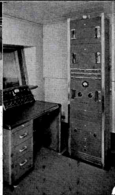
New Studio Control Room
